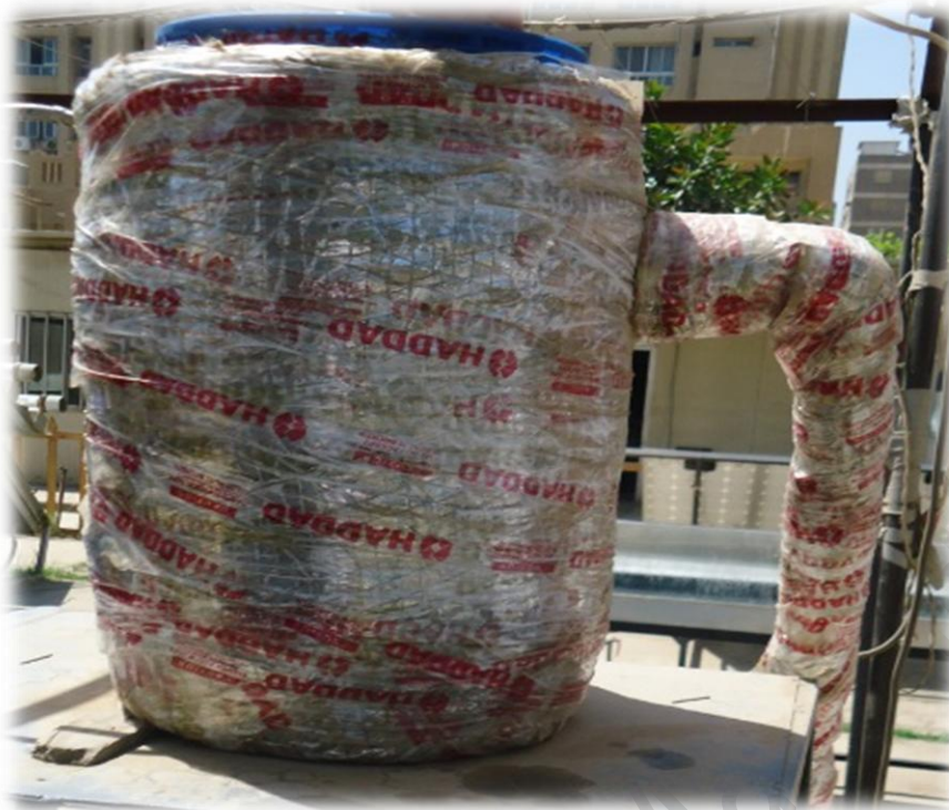
Fig 3.11 insulated storage tank
